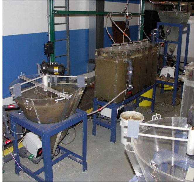
Fig 1. Photograph of the pilot-scale AST system. Right/rear: Primary clarifier; middle: aeration basin; left/front: secondary clarifier.
