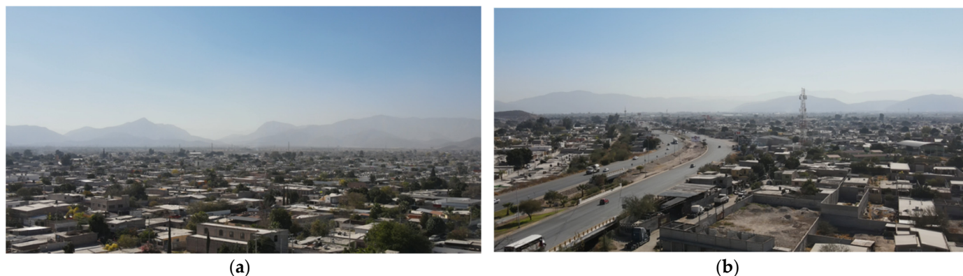
Figure 16. Aerial views of the city of Gomez Palacio, Durango taken by DJI Mavic Air 2 UAV at an altitude of 100 m; (a) Periferico zone, 23 September, (b) Periferico zone, 27 September.
