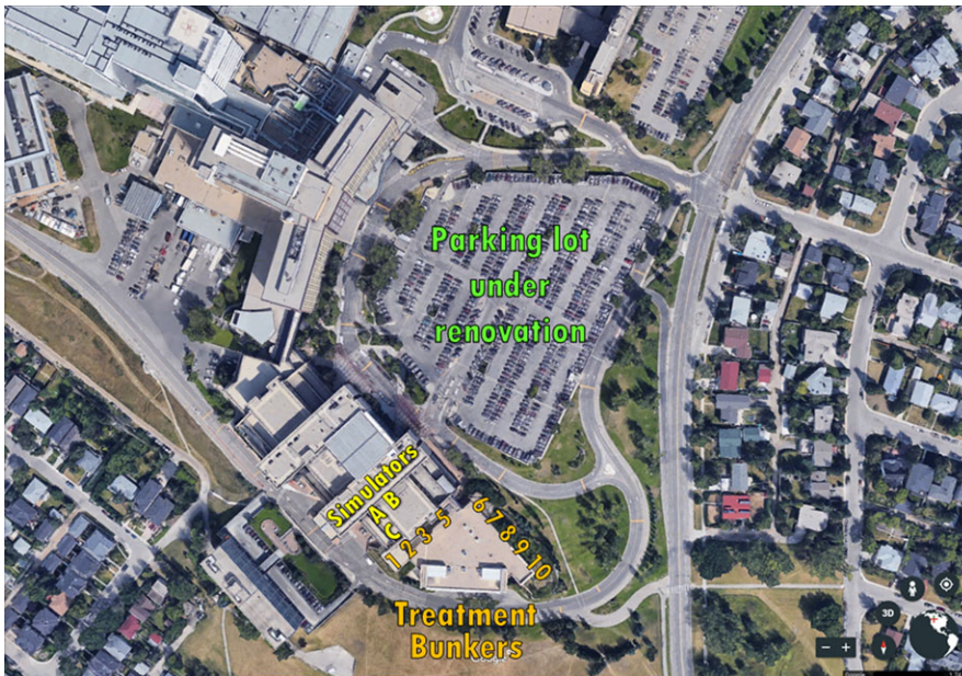
FIG. 1. Location of construction site relative to TBCC. Treatment vaults are labeled numerically. The stereotactic radiosurgery (SRS) vault is #3. The location of the CT and conventional simulators is also indicated.
