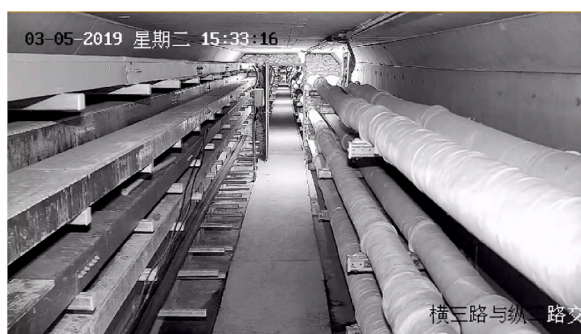
Fig. 7. Interior environment of the utility tunnel used for experimental case study.
