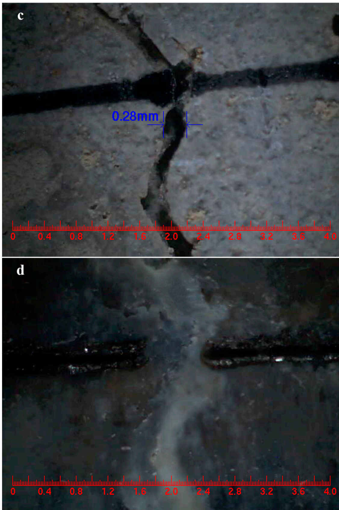
Figure 19. Self-healing of surface cracks in mortar. (a) Control mortar, (b) control mortar after three days of self-healing, (c) mortar containing microcapsules, (d) mortar containing microcapsules after three days of self-healing.
