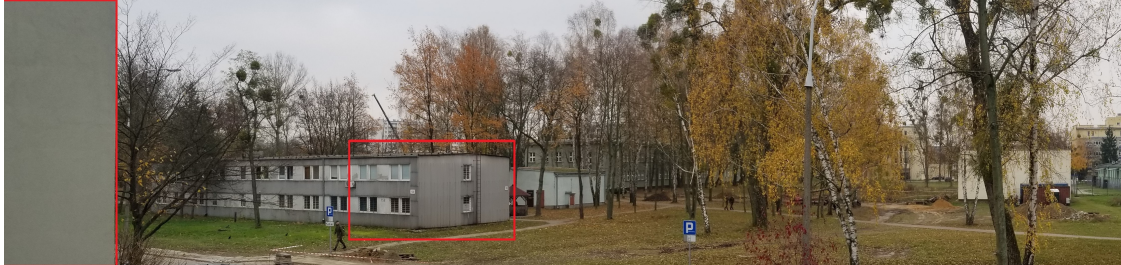
Figure 17. Panoramic picture of the Test Area 1.
