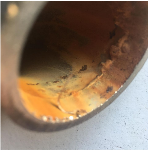
Fig. 3 Welding section after six years of use of inox AISI 316L piping ring. It is possible to note fusion defects by hot weld cracking. This problem was found in three dialysis centers after the removal of the stainless steel and its replacement with PEX
