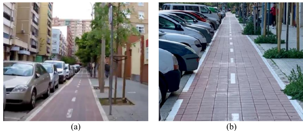
Figure 6. Sidepath without physical or vegetated curb next to parked motorized vehicles: (a) parallel parking, and (b) perpendicular parking.
