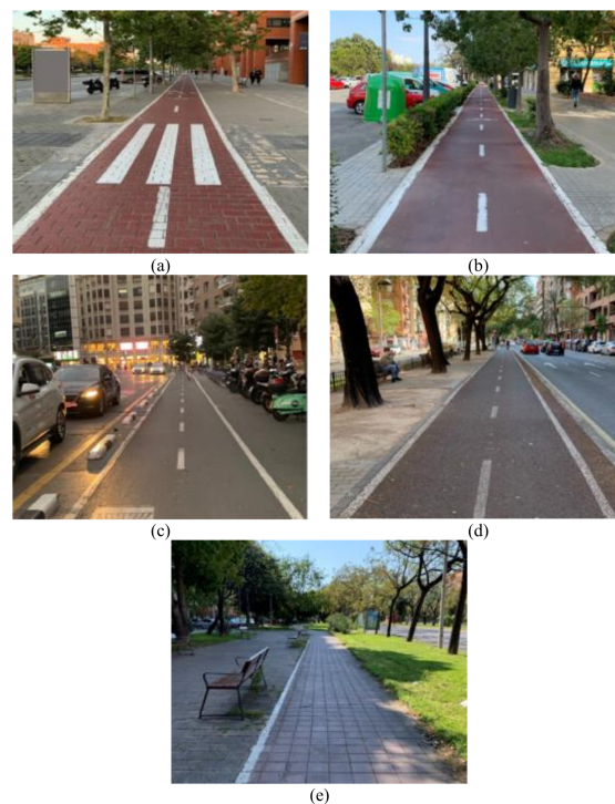
Figure 1. Typologies of bicycle tracks: (a) sidepath without physical or vegetated curb, (b) sidepath with vegetated curb, (c) protected bicycle track, (d) sidepath on median next to motorised traffic, and (e) sidepath on median.
