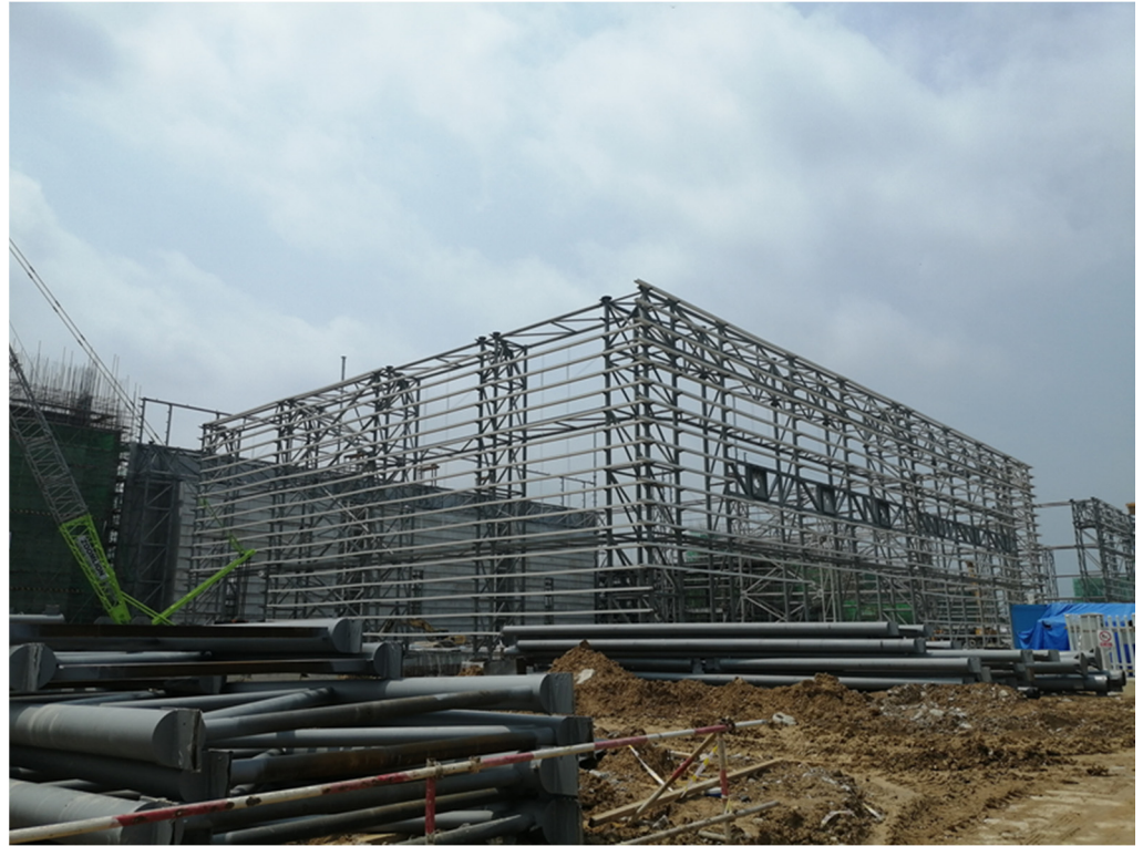
Figure 1. Converter station steel structure site.
