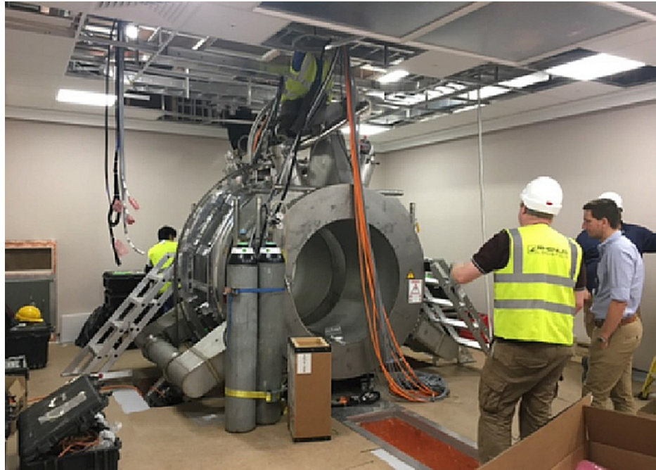
FIGURE 1: Installation of the MRIDian bore
