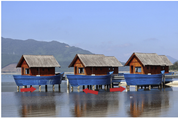
Fig 9. The concept of this new technique originates from river houses built on stilts (red arrows) (commonly found in Asia) that allow a strong fixation of residential structures, against large external forces, such as floods.
