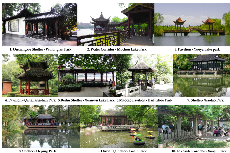
Figure 3. Photos of the 10 amenity buildings included in the study.
