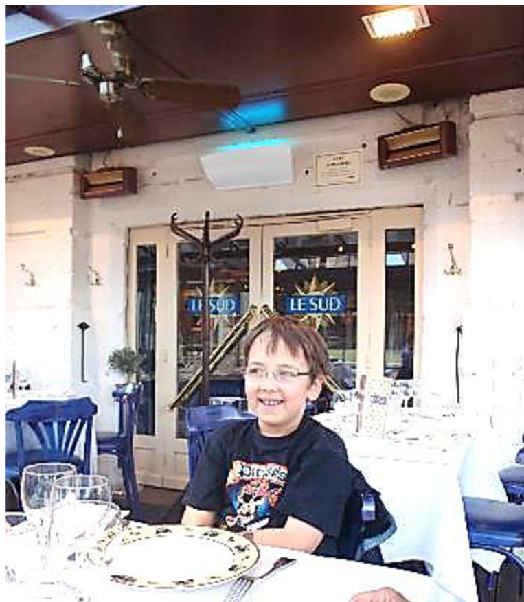
Figure 2. UV light trap mounted high above restaurant entry doors tends to attract flies to the doors with possible entry inside building, Lyon, France.
