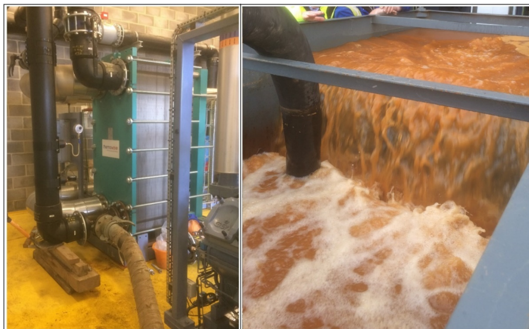
Figure 6. Recirculation of citric acid solution through the plate heat exchanger at Abbotsford Road, (left), to remove accumulated ochre (which can be seen in the recirculation tank, (right)). Photos reproduced with permission of © David Banks, after [2,36].
