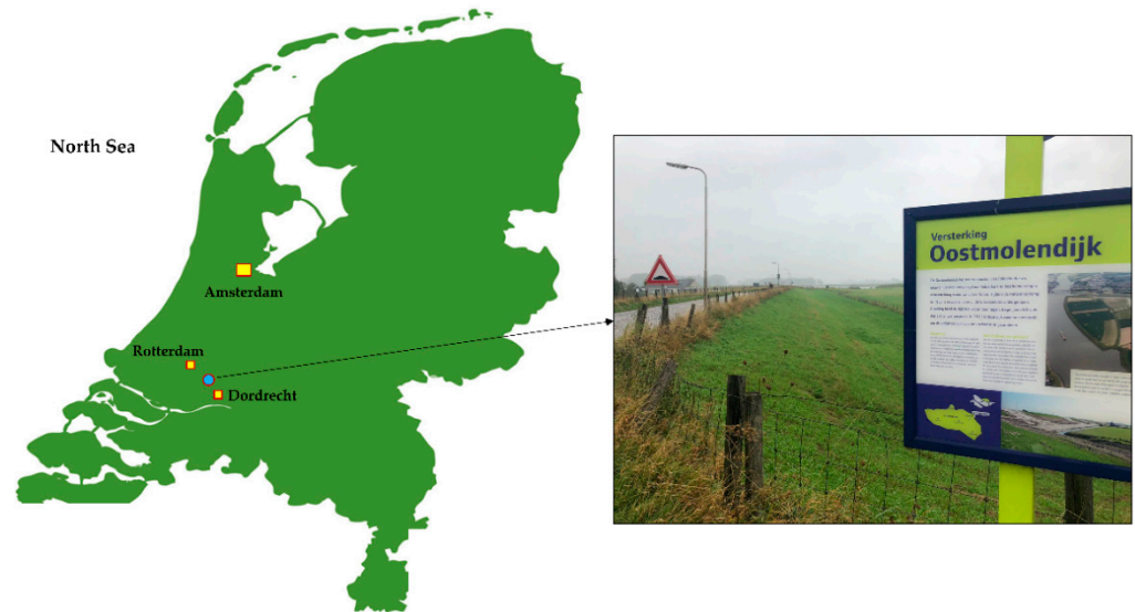
Figure 7. Location of the case study embankment Oostmolendijk.
