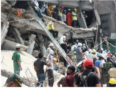
FIGURE 4: Rescue at Rana Plaza collapse.
