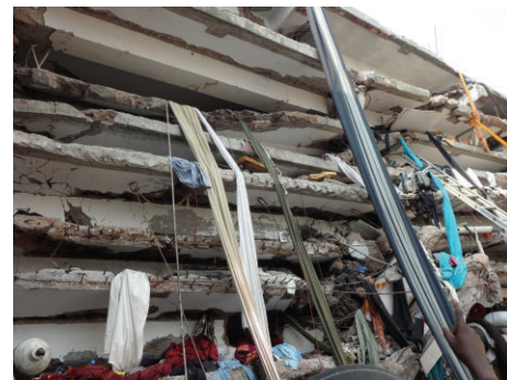
FIGURE 3: What happened after Rana Plaza collapsed.
