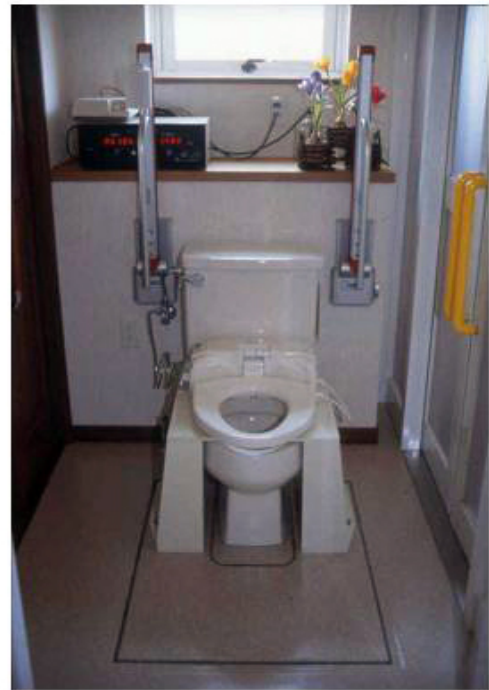
Fig. (5). Toilet weight-monitoring system.
