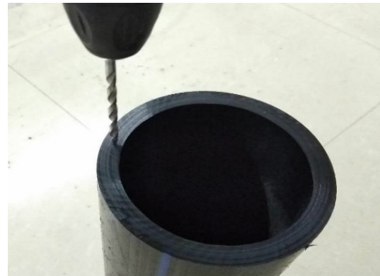
(b) Drilling holes
