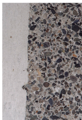
Figure 3. View of a deactivated decorative concrete slab with a binder composed of 80% glass powder and 20% CEM I 52.5 R cement. The left side of this photograph shows the appearance of the concrete before applying the chemical or mechanical treatment.
