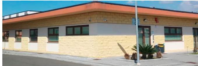
Figure 23. Technological pole building.
