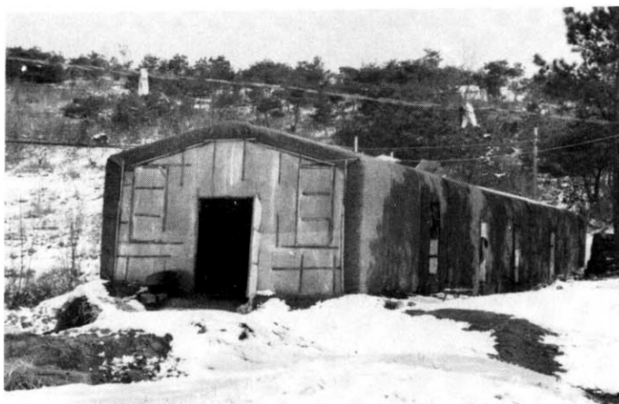
Fig. 1. The cultivation house was almost totally enclosed with a thick wall to protect from direct sunlight and to insulate in order to maintain a temperature of 15~20°C.
