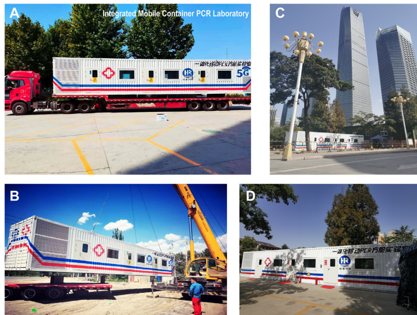
Fig. 1. The IMCPL units in China. (A) An IMCPL unit loaded onto a truck and later transported to Korla, Xinjiang. (B) An IMCPL unit being unloaded from the truck and installed locally. (C) An IMCPL unit set up at the Hongkong West Road in Qingdao, Shandong, next to the buildings of Guoxin Haitian Center. (D) An IMCPL unit installed at the Qingdao Navy Special Service Sanatorium, Qingdao, Shandong.
