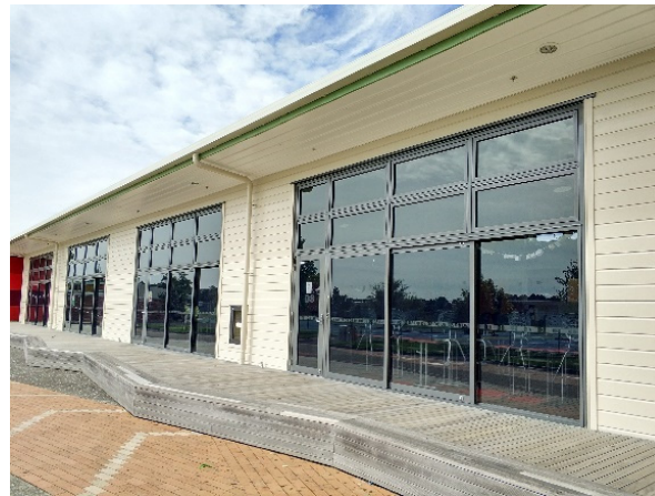
Figure 2. Retrofit school building.
