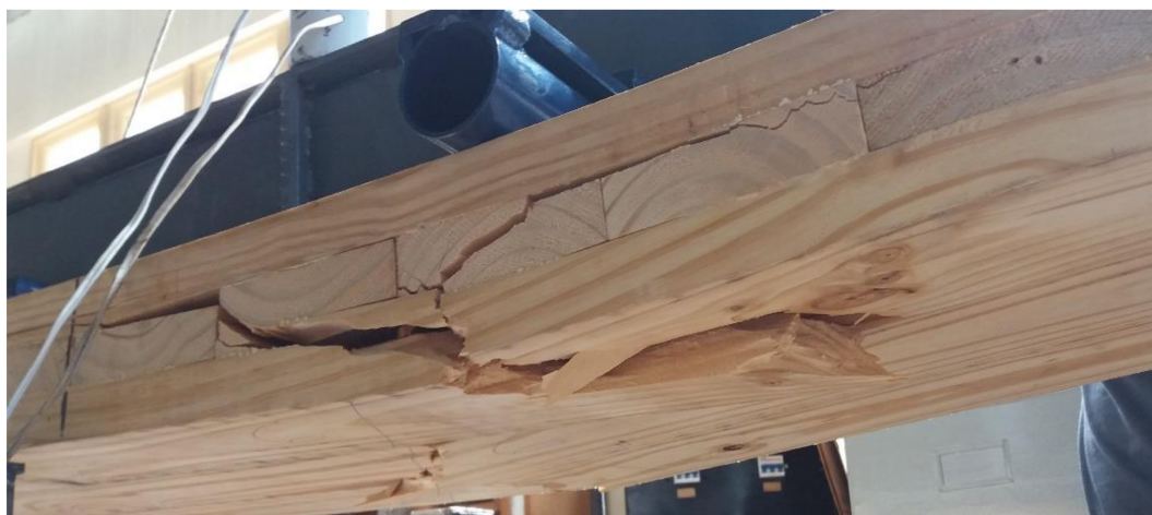
Figure 6. Tensile failure on the bottom of the CLT followed by rolling shear failure.
