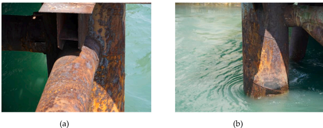
Fig. 5. Example of image data acquisition at construction site: (a) Site image sample 1; (b) Site image sample 2.
