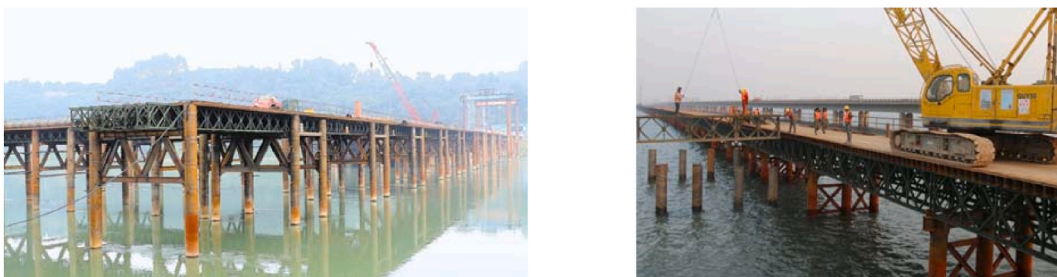
Fig. 1. Example of offshore construction wharf.
