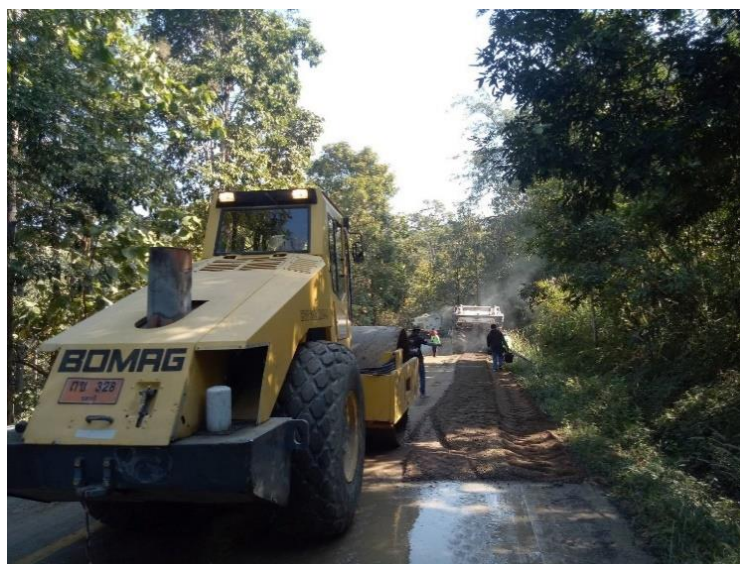
Figure 2. Possible application using AAM for in situ pavement recycling, Mae Hong Son province, Northern Thailand (author).
