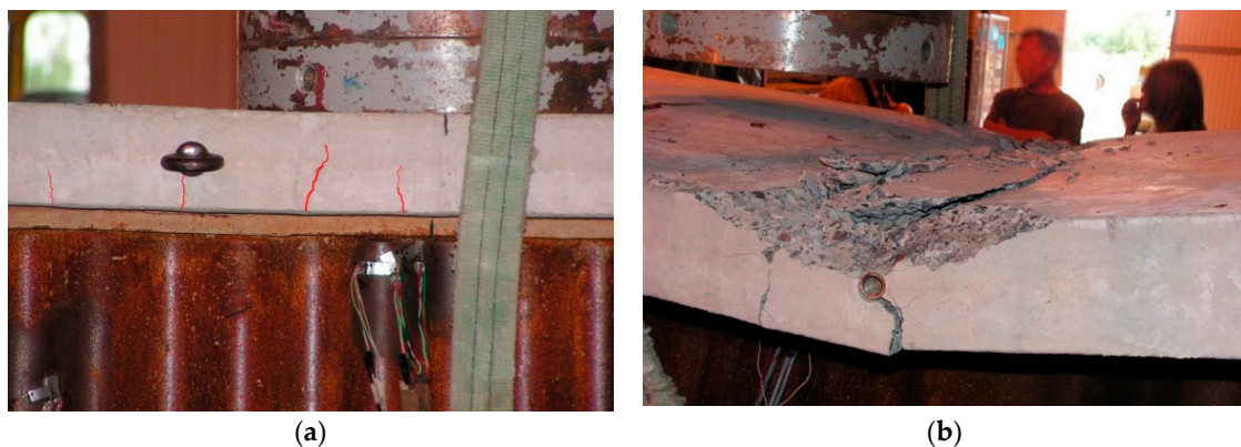
Figure 7. Reinforced concrete slab damage: (a) Crack morphology; (b) concrete crushing.
