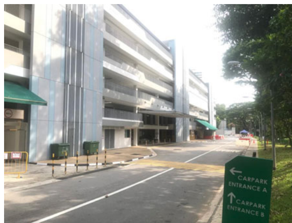
Multi-story Carpark (MCSF).
