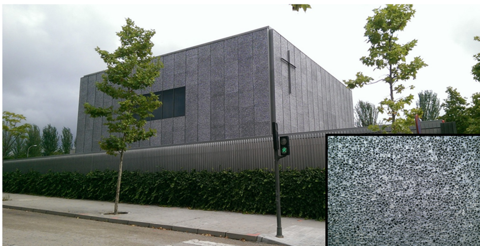
Figure 15. Protestant church in Terrasa, Spain, clad with Alusion foam. The inset shows a detailed view of the foam structure (courtesy of John Banhart).
