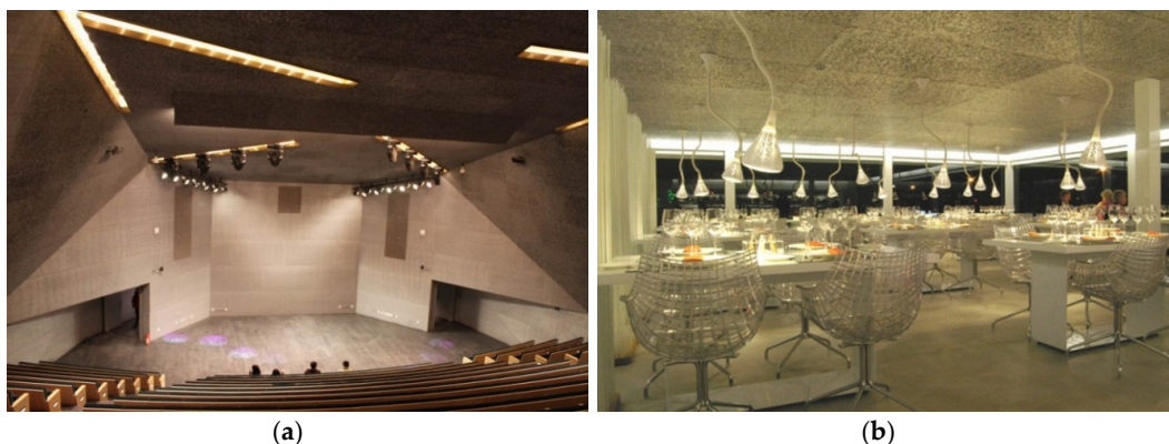
Figure 10. Ceiling of (a) audience hall; and (b) restaurant covered by Alusion foam for sound control (courtesy of Cymat).
