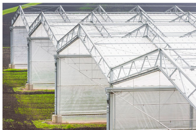
Figure A2 Closed shelters and panels of the future climate plots of the GCEF, photograph taken by UFZ/ André Künzelmann
