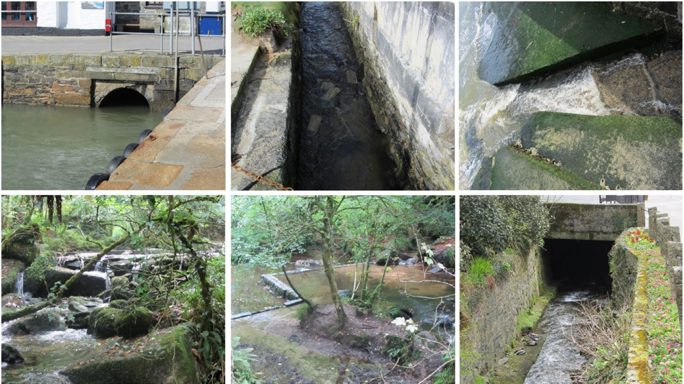
FIGURE A4 Examples of barriers in four streams in south Cornwall. Clockwise from top left: the mouth of the Mevagissey Stream; a canalised section of the Portmellon stream; the mouth of the Portmellon stream; the Polperro flowing through one of several culverts in Polperro village; heavily silted impounded section of the Kennall River at the Kennall Vale gunpowder works; barrier to upstream movement of trout, Kennall Vale.
