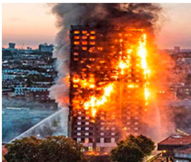
Figure 1. Burning Grenfell Tower at the height of conflagration; the black smoke at the top is combustible material burning without water; the whitish gas is mainly alumina dust from the reaction of Al and or Al_4C_3 and steam, as the water still being applied. Note the intensity of the conflagration where the water hits the building, and the associated whitish clouds around.
