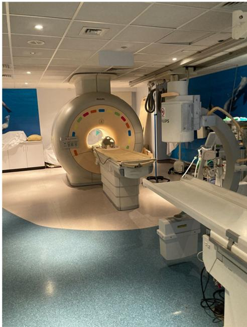
**Fig. 2** X-ray and CMR (XMR) room. XMR room with the x-ray and MR equipment joined by a movable tabletop. The c-arm of the x-ray unit is seen in the right side and the 5-gauss area is demarcated by a change in the floor colouring from the MR to the x-ray end of the room
