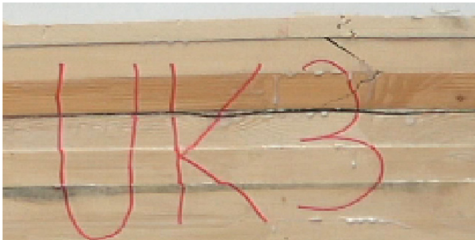
Figure 4. Failure of joint in beam-type UK.
