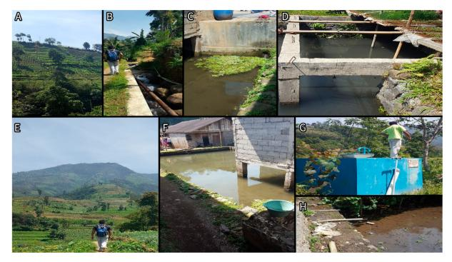
**Figure 4.** Flow of water in Topengan. (**A**,**E**)—Surrounding environment of Topengan village. (**B**)—Pipes from the spring to the holding tank. (**C**)—Concrete outflow channel to the fishpond. (**D**)—Crops grown above the fishpond. (**F**,**H**)—Fishpond. (**G**)—Water holding tank.
