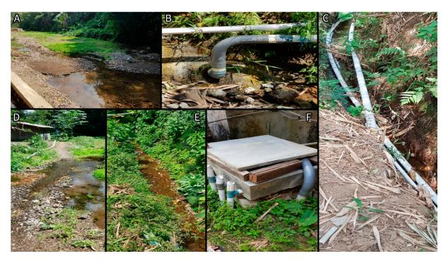
**Figure 3.** Flow of water in Losari. (**A**,**D**,**E**)—Neighboring environment of groundwater spring. (**B**,**C**)—Pipes from spring to holding tank. (**F**)—Water holding tank.
