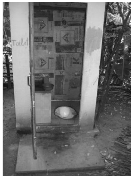
Figure 1 Pour-flush latrine in Beung village of Kompong Thom province, Cambodia. The pictured latrine features a tiled cement slab with a ceramic bowl, a cement water basin and a plastic ladle for anal cleansing.
