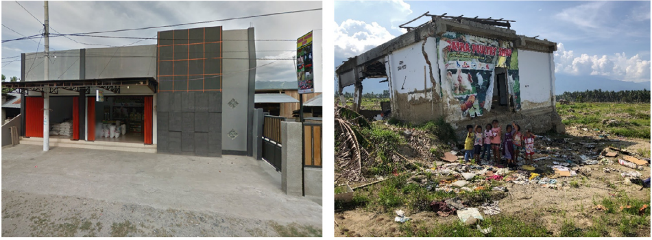
Fig. 10. Patra Poultry Shop in Jono Oge from (left) before the earthquake in Google Streetview and (right) after the earthquake as observed by the reconnaissance team. The children's faces in the photograph taken by the reconnaissance team are blurred to protect their privacy.
