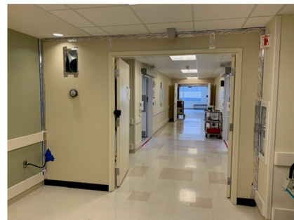
FIGURE 2 Anteroom is shown after the construction. Doors were closed in panel A, whereas panel B shows the anteroom doors open, facing the hallway
