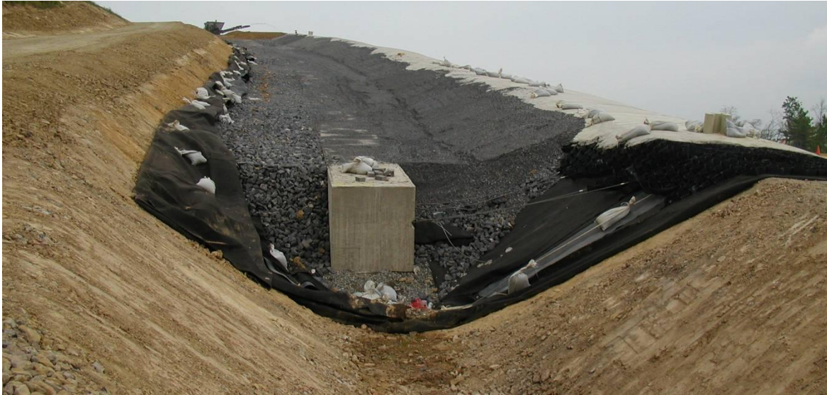
Figure 14. Photo showing cross section of concrete deadman anchor system.
