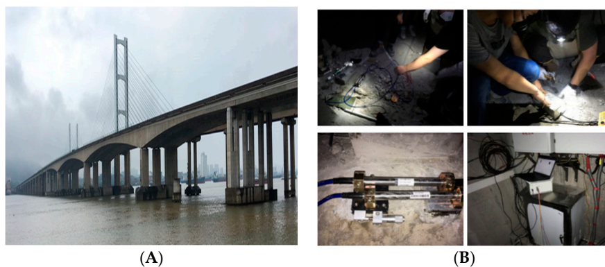
Figure 4. Test verification of Jiujiang Bridge. (A) Jiujiang Bridge, (B) Test process.
