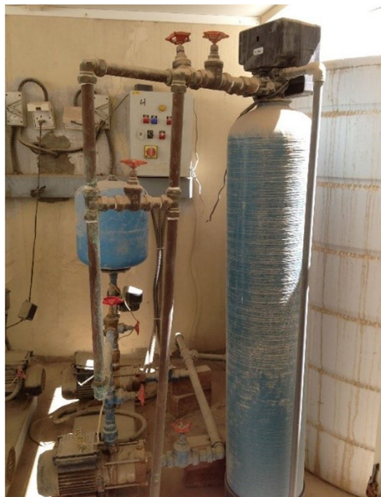
Figure 2. Typical point-of-entry filtering system (Lavender Village residence), Doha.
