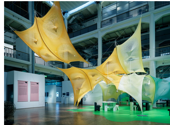
Fig. 3 Zoirotia at ZKM, Germany. Colour is controlled by grading the duotone system of Jacquard knit. The grading of intensity follows the structural performance as material extensions around the pre-tension points grade translucency. CITA 2022
