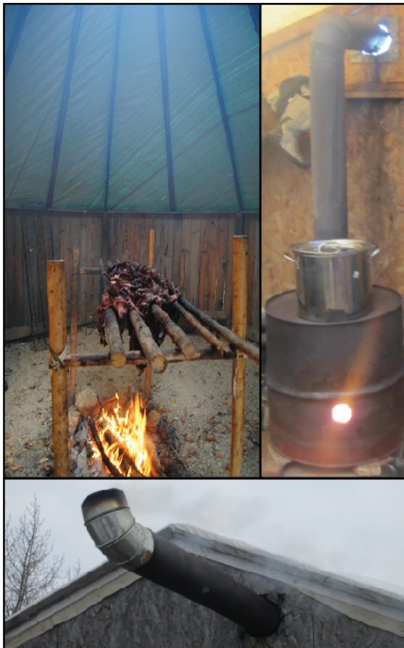
Figure 2. Clockwise from top left: Figure 2(a). Geese being smoked over a fire in a traditional game-smoking tent. Smoke is clearly visible towards the top of the photo. Figure 2(b). A wood burning wood stove made of a steel 45-gallon drum in a hunting cabin. Figure 2(c). A chimney flue exiting a hunting cabin. Photo permissions: R. Moriarity (2a) and M.Wilton (2b and c).
