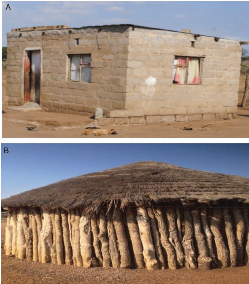
Figure 1. Examples of high- and low-quality homes. (A) High-quality housing with cement block internal and external walls, some screened windows, and metal roofing. (B) Low-quality housing with stick walls, grass roofing, and no windows.
