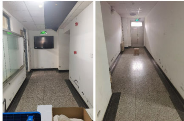
Figure 18. “L” shaped long corridor.
