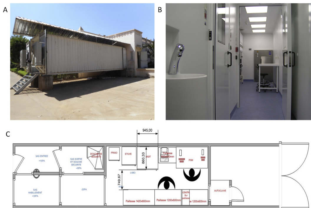
FIG. 1. (A) Exterior view, (B) interior view and (C) blueprint of CICM BSL3 laboratory. BSL3, biosafety level 3; CICM, Charles Mérieux Center for Infectious Disease.
