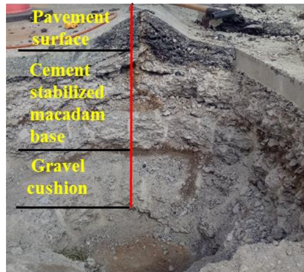
Figure 1. Pavement structure at the arch expansion section.
