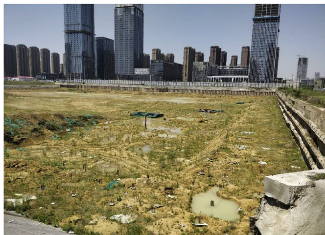
Fig. 2. Status of foundation pit.
