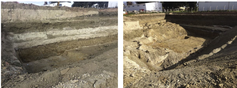
Fig. 11. Excavation area site 2 (courtesy of CMP).
