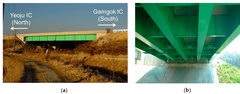
Figure 3. (a) Front view and (b) bottom view of Samseung Bridge, Korea.
